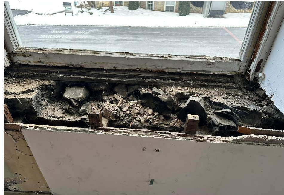
1908 BUILDING - WINDOW SILL
