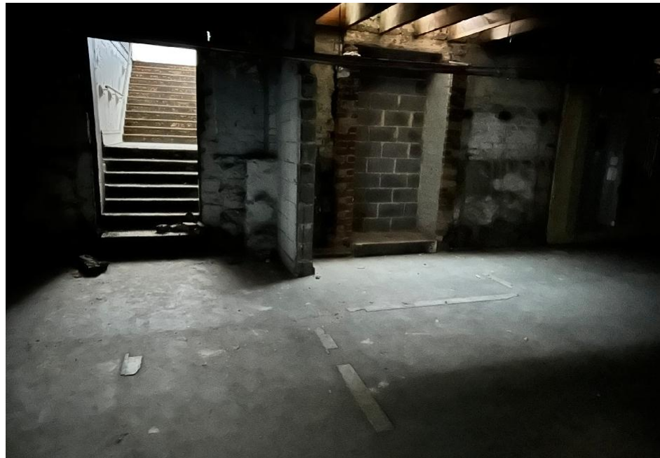
1879 BUILDING / STAIRS OF 1908 BUILDING
